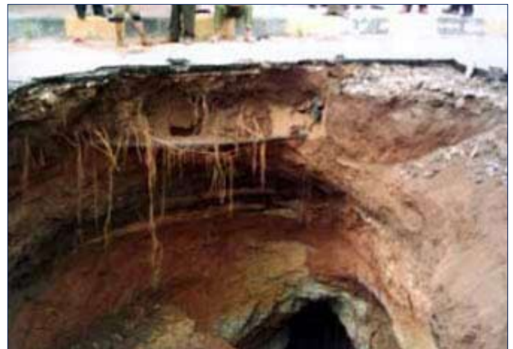
Once drained, the sinkhole revealed marl and limestone, and what may be an ancient tunnel. (Photo: Kholoud Mahamed Ali)
