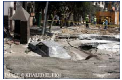
Water-filled sinkhole in Old Cairo destroys a car.
